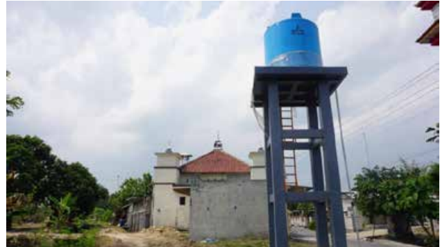
Water tanks for Karangmalang and Craken Villages in Indonesia
